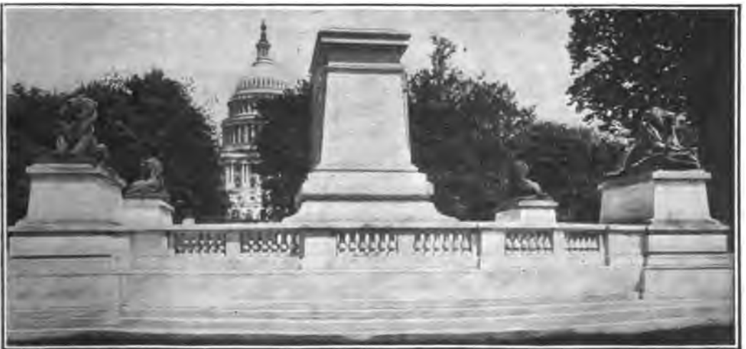
Photograph by Commercial Photo Co., Inc., Washington, D. C.
